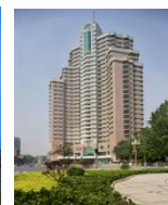
Somerset Olympic Tower Property Tianjin
