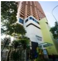
Somerset Liang Court Property
