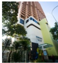
Somerset Liang Court Property
